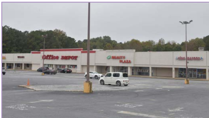
Figure 1: Many older strip-center developments, such as this plaza along Memorial Dr, are declining and in need of redevelopment
