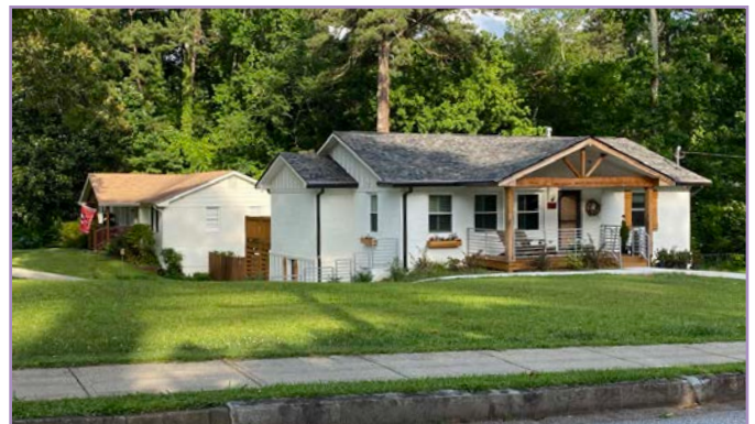
Figure 9: Older homes in established neighborhoods offer more affordable quality housing options for residents, compared to new construction
